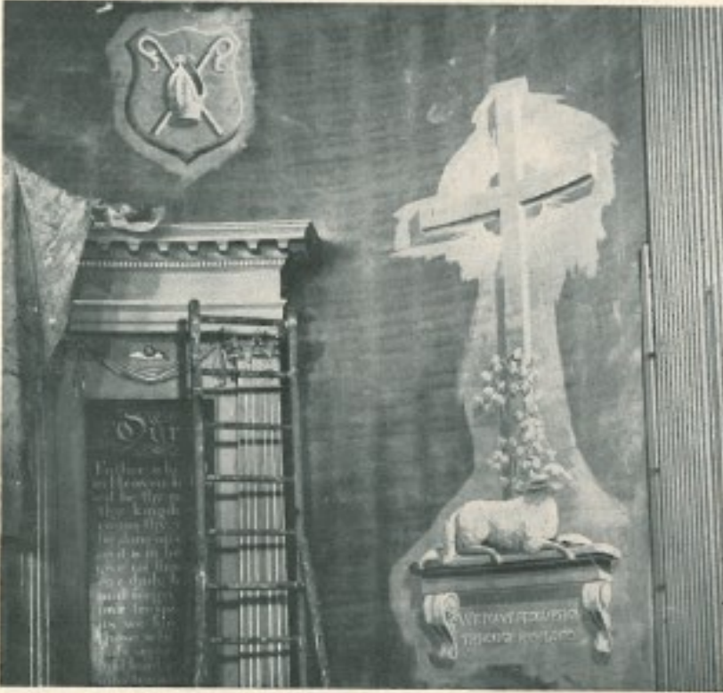
THIS CLOSEUP clearly shows the contrast between the restored portion and that still to be cleaned. When this photo was taken only the two designs had been touched.
